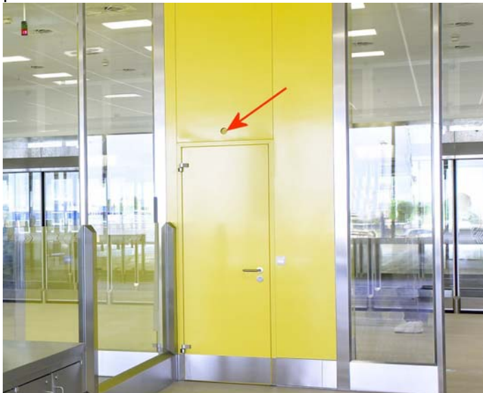
Picture 4: Clean Room wall with hole for overflow (arrow)
