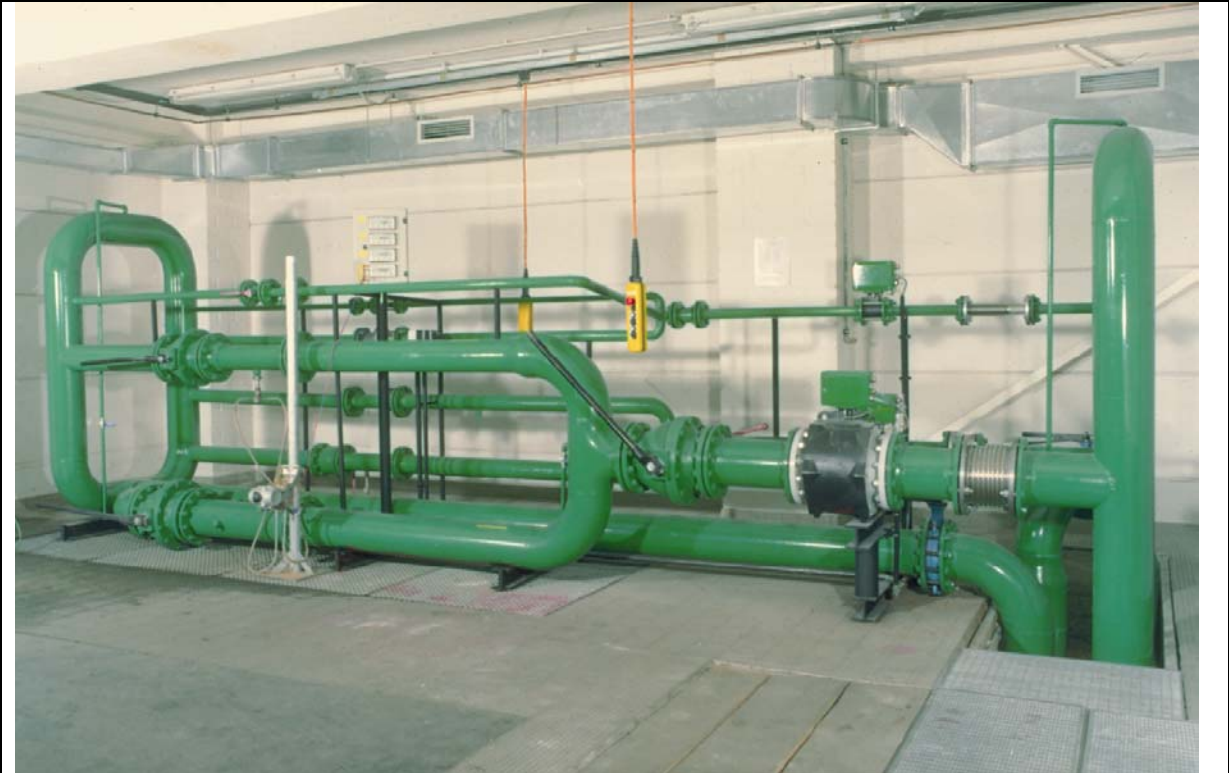
Fig. 10.1: Manufacturer’s water calibration rig for pipe sizes 0.5 through 12 inches, max volumetric flow 400 m 3 /h (1760 GPM).
