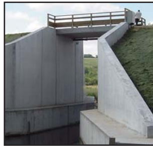
Control sluice built according the scale model conclusions
