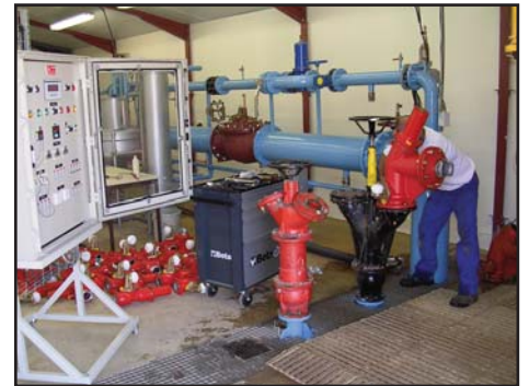
Hydraulic testing of irrigation hydrant
