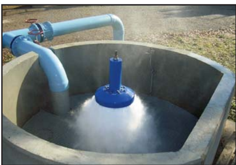
Plotting of discharge-pressure curve for a ND200 relief valve calibrated at 2 bars discharging up to 750 l/s
