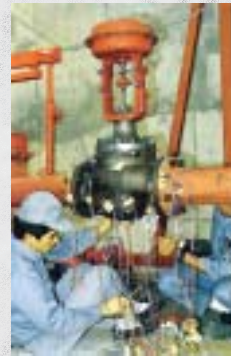
Piping stress test
