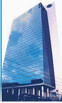
Installed savic-net™ EV integrated building automation system
