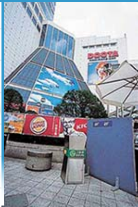
Installed electronic air cleaner for smoking areas
