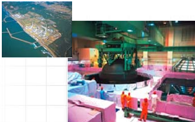
Switches for Safety in a Nuclear Power Plant Tokyo Electric Power Company Kashiwazaki-Kariwa nuclear power plant
